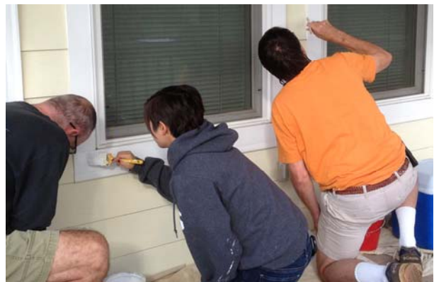
Volunteers paint the trim on the front of the house.
